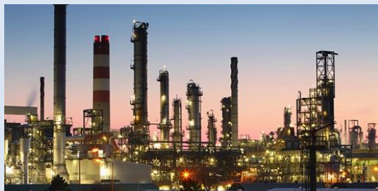
Down-hole power supplies (gas & oil)
