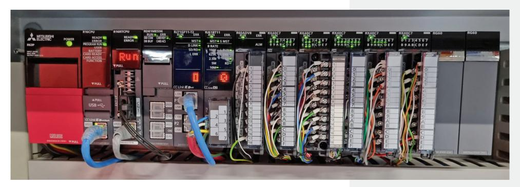
Automation on the Harwin assembly line: Power supply, PLC, communications and input modules
